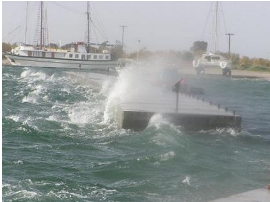
Fig. 166 FDN's concrete U-block floating breakwater applied for wave heights up to 2m (90% damping can be achieved).
