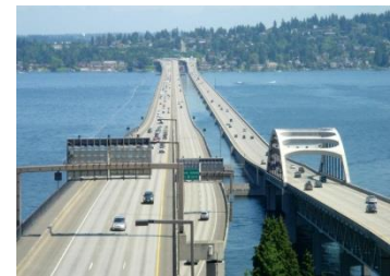
Fig. 30 Murrow Memorial Floating Bridge, USA [6].
