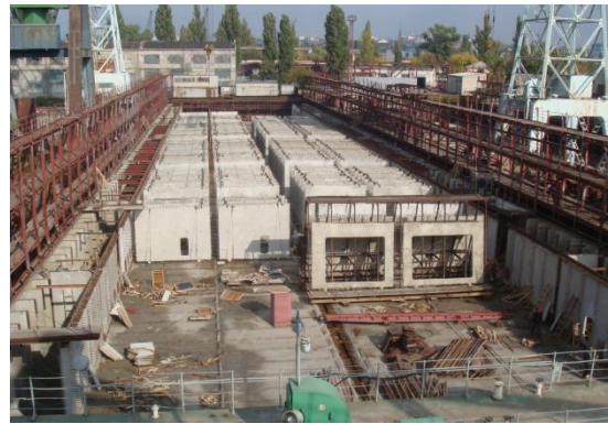
Fig.19 Impression (left) from research of a building with a height of 60m on a floating base of 90m by 90m and (right) construction of a floating base of 45m by 245m from pre-fabricated elements in a floating dock.
