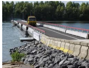
Fig. 26 Floating road, Hedel, The Netherlands [5]; the floating element are made from aluminium, but concrete is an option.
