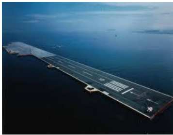
Fig. 2519 Mega-float airfield, Tokyo, Japan [3].
